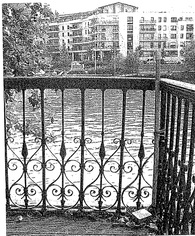
Balustrade du balcon Fournaise (Photo J.-C.B.)
